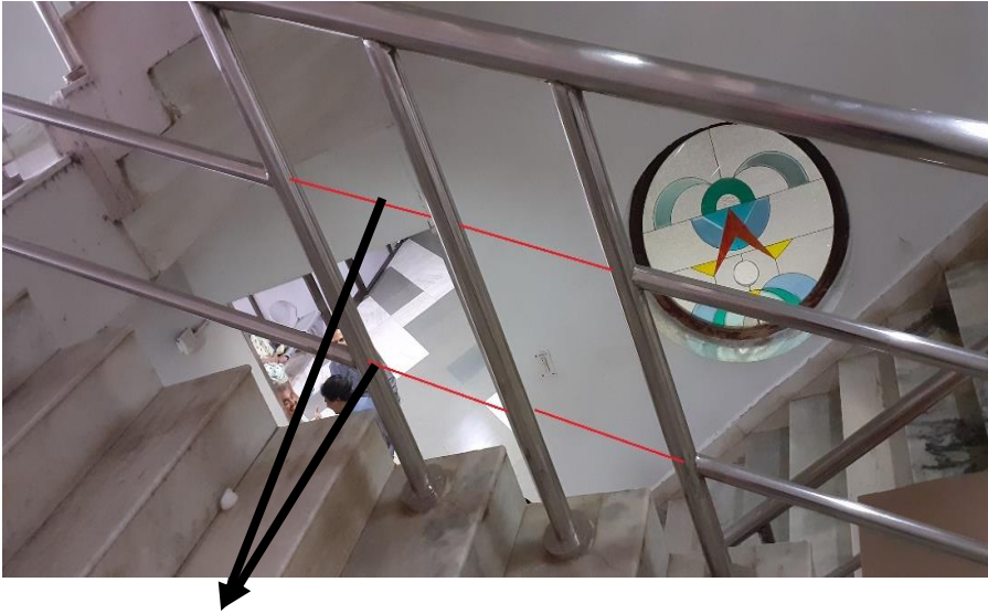
Additional SS pipe in mid of hand rail CRC Main Staircase
