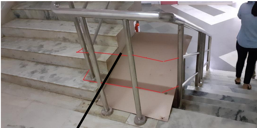
Additional SS pipe at Corner of hand rail CRC Main Staircase
